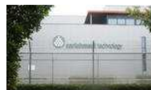
The enrichment facility in Almelo has a long story.
