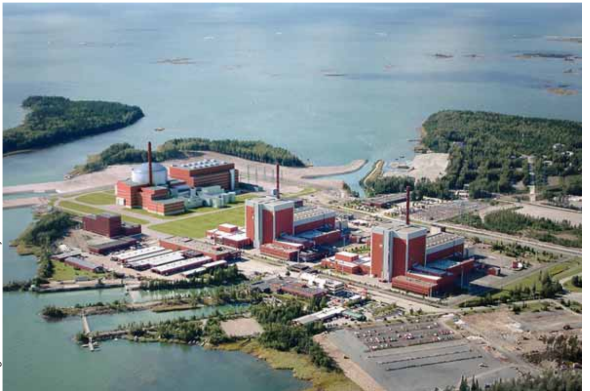
A vision of the Olkiluoto 3 reactor (montaged nearest to the sea).
